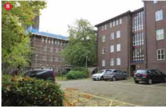
View of the entrance forecourt to Building 10
