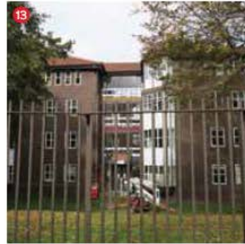
View of the southern entrance to Building 10
