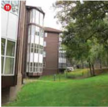
View of the southern landscaped bank
