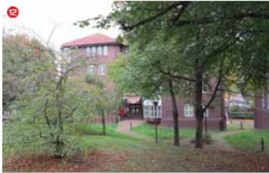
View of the landscaped zone to the south of Building 11
