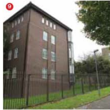
View of Building 11 from the north west
