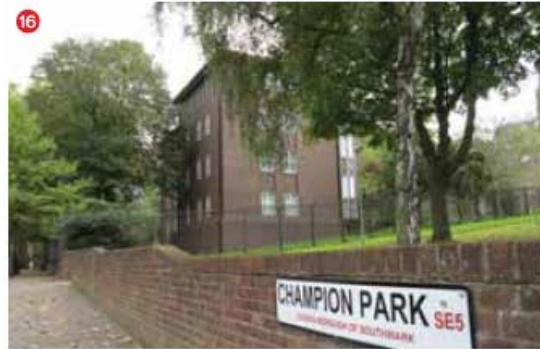
View of Building 11 from the north west
