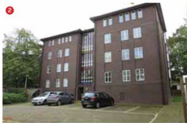
View of Building 10 from the north
