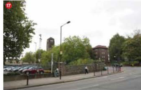
View of Building 11 and the listed tower from Denmark Hill / the north west
