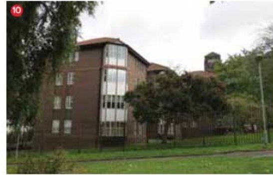
View of Building 11 from the west
