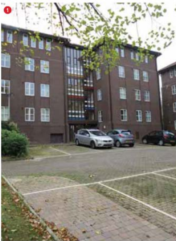
View of the entrance forecourt to Building 10
